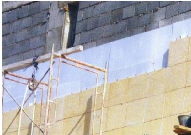
figure (8): External insulation system
