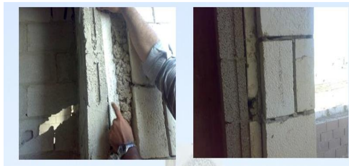
figure (7): Building a wall between them thermal insulation panels
